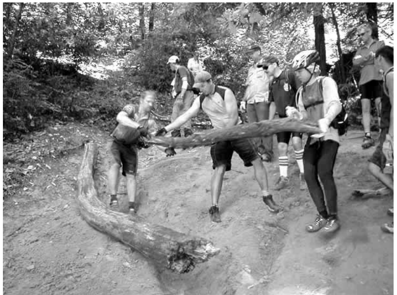
Then crews reinforced the downhill sides of the trenches with dead wood.
