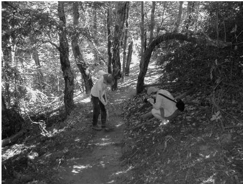
Other crews put final touches on the bypass of the steep section
