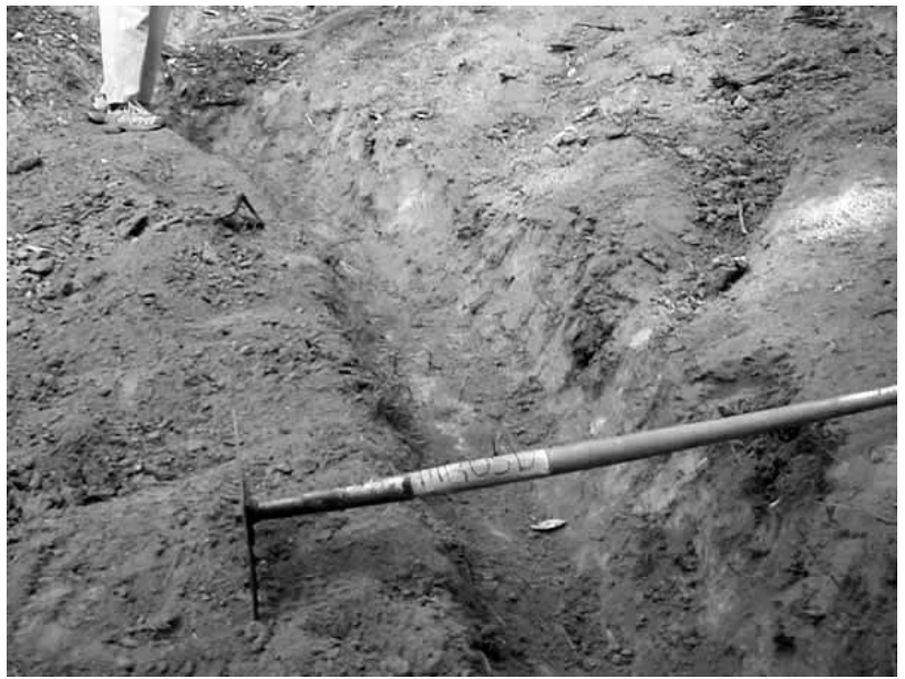
First, work crews dug trenches divert water off the old skid-road trail.
