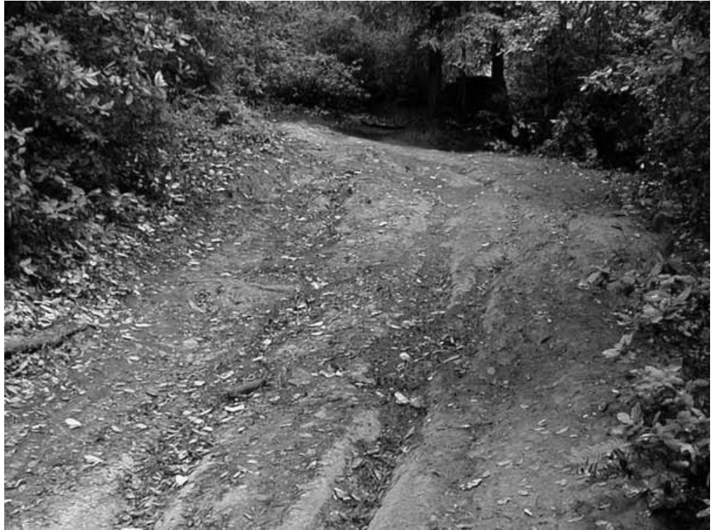
The steep eroded section of the old blue blossom trail dumped sedimentation in to the creeks of ECDM.
