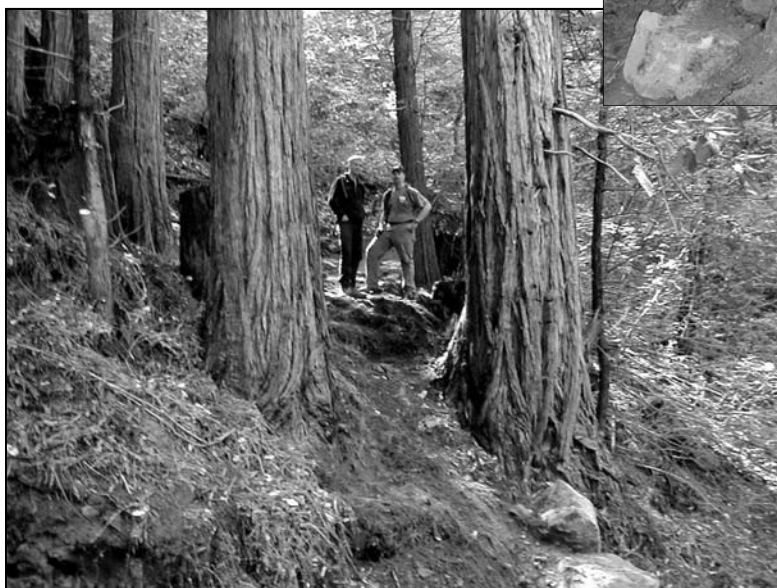
The Goalposts During. Some of the rocks have been moved by the mini excavator, and the approach to the drop through the redwoods has been roughed in.
