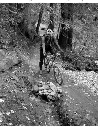
of a small French drain where a spring flows out of the side of the hill. To build a French Drain, dirt is removed where the water is flowing, and rocks are put back in their place, then a layer of dirt is piled on top to provide a dirt surface. The space between the rocks allows the water to flow between them.
